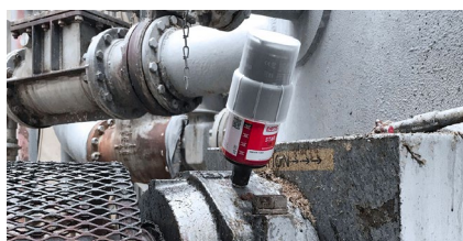
Lubrication of a pillow block bearing on a blower
