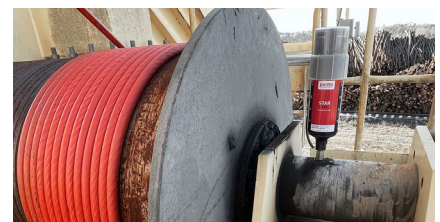
Lubrication of a crane cable pulley bearing
