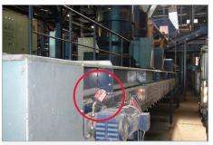
Lubrication of flange bearing on a conveyor
