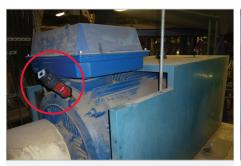
Lubrication of pump motor
