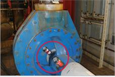
Lubrication of drive shaft on a pump
